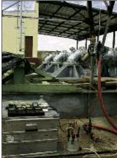
**View over the head of No. 2 shaft of the abandoned Berg Aukas Mine: Four strong submersible pumps of which each has a capacity of 360 m<sup>3</sup>/h were installed in the shaft in 1997 to lift groundwater from the open underground mine workings and the dolomitic host rock. The four pumps can be run simultaneously, but presently the set-up is two production pumps and one stand-by pump.**
